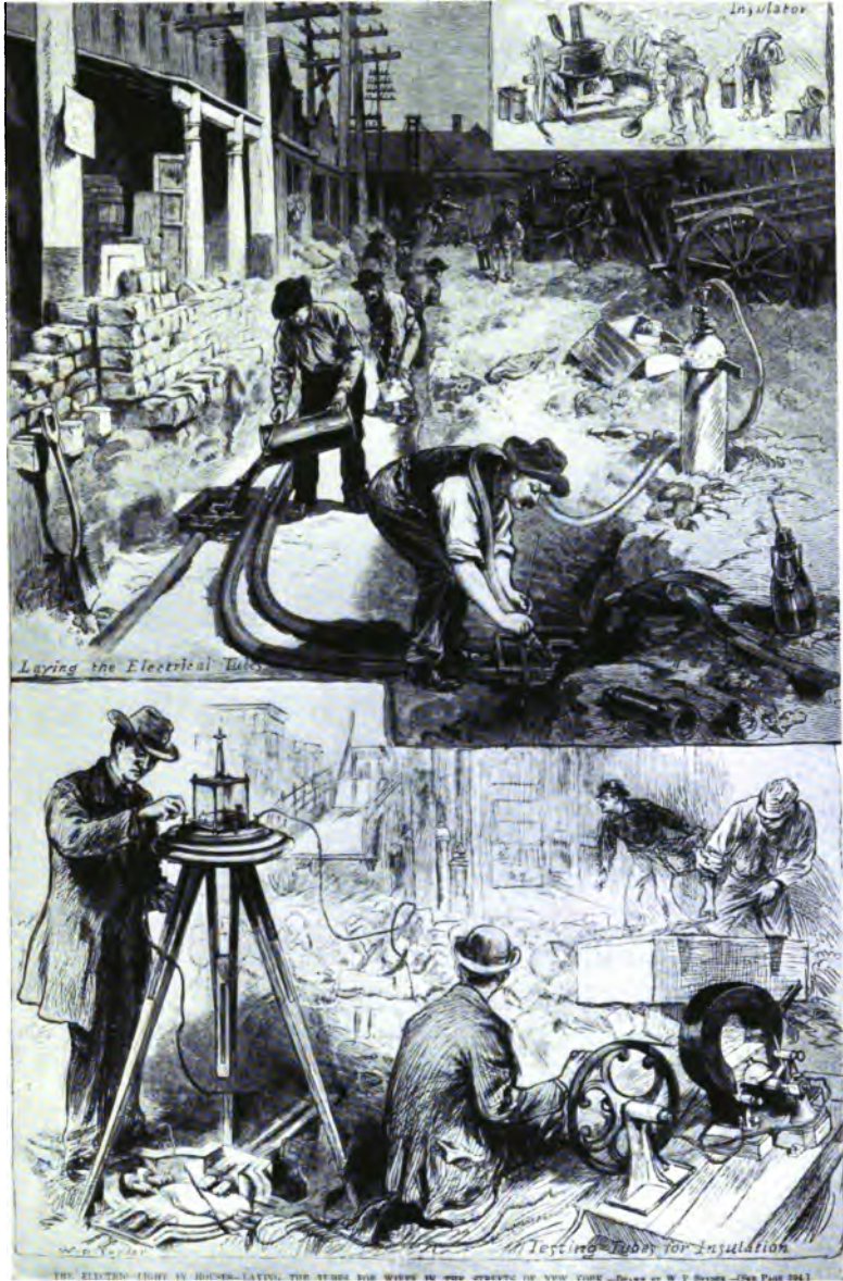
THE ELECTRIC LIGHT IN HOUSES Laying the tubes for wires in the streets of New York Drawn by W P Snyder, Harper's Weekly , 1882
